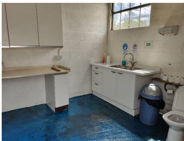
This is what the toilet looks like.
